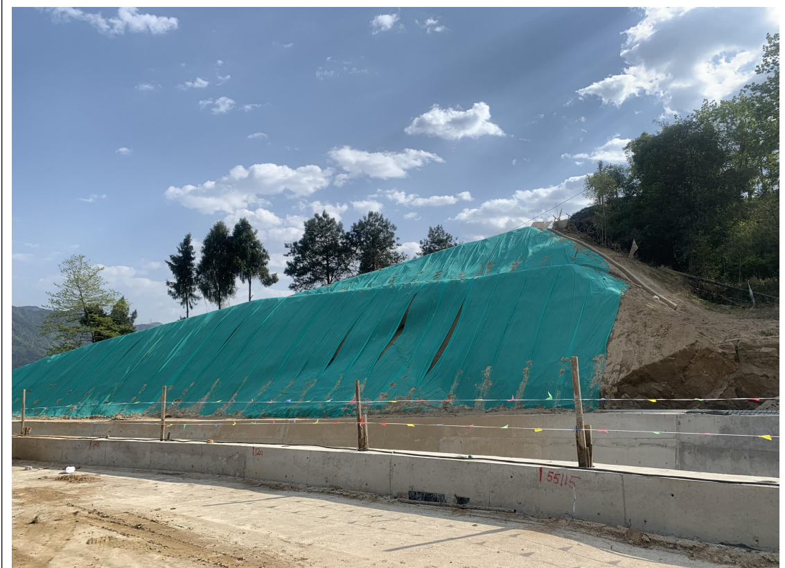
边坡临时苫盖
