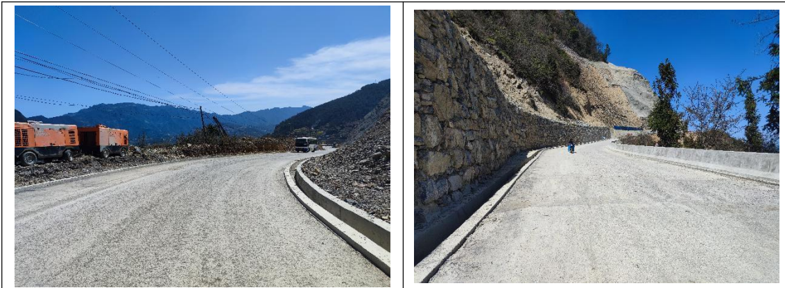
K6+440~K6+940 路基水稳垫层铺筑
