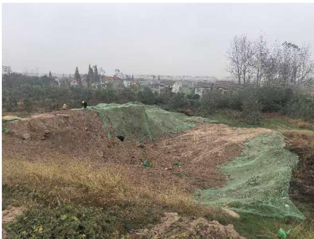
临时堆土临时苫盖
